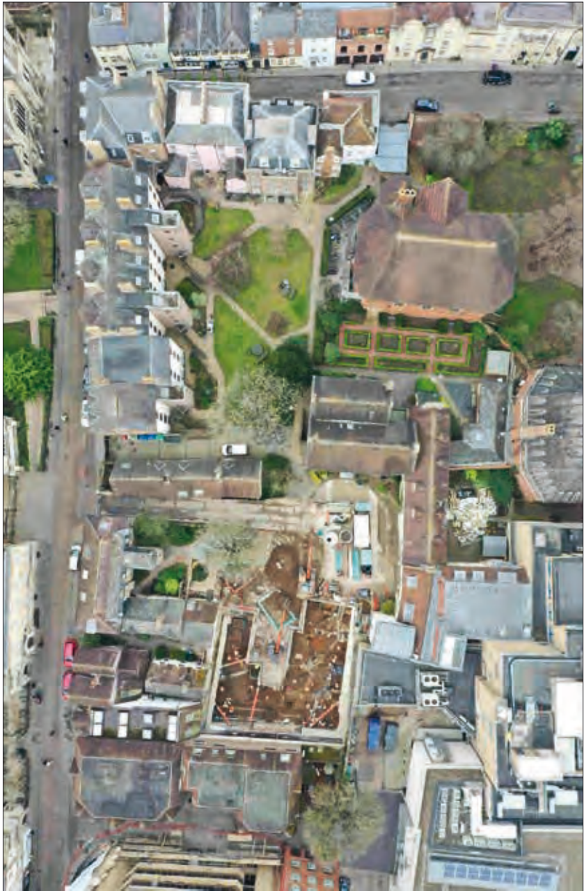
An aerial view of the Frewin site redevelopment work, February 2022
